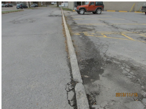
Building Condition Assessment for The Town of Mississippi Mills
