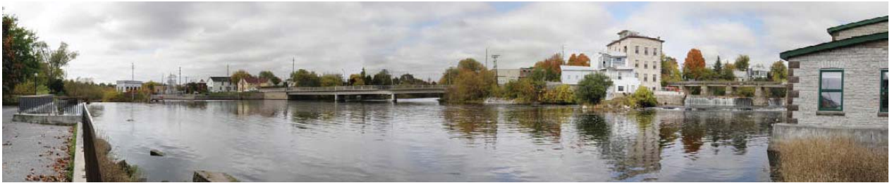
Mill pond above No. 2 falls, from the Riverwalk. Industrial buildings, bridges and residential buildings terminate the viewplane.
