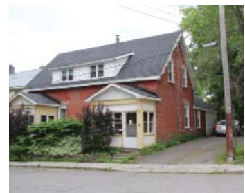
Example of Ontario Vernacular on Union Street South.
