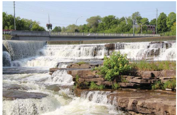
The flow of water over weirs, rock ledges and falls is a character-defining attribute that shall be conserved.
