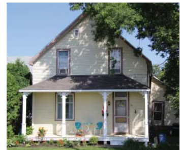
Worker's cottage style, finished with horizontal siding, Main Street West.
