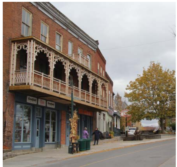
Documentary evidence, such as historic photographs, may be used to accurately reproduce missing elements like porches.
