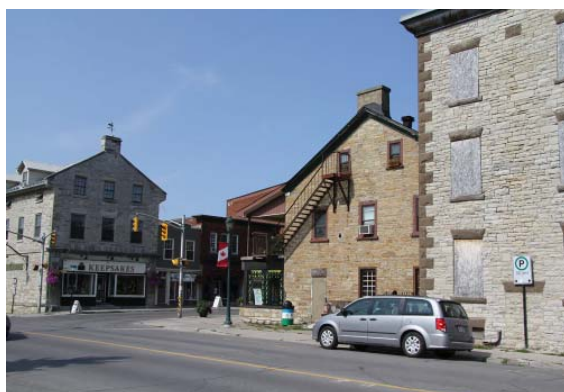
Several stone buildings anchor the intersection of Bridge and Mill Streets, and define the character of this area.
