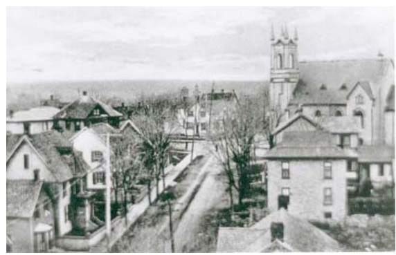
Union Street South, with Trinity Methodist Church and Main Street East in the background. The street continues to be characterized by a predominantly residential character and the presence of low garden walls and street trees. Source: Michael Dunn collection. N.d.
