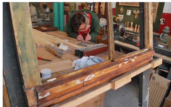
Historic window being repaired at a millwork shop.
