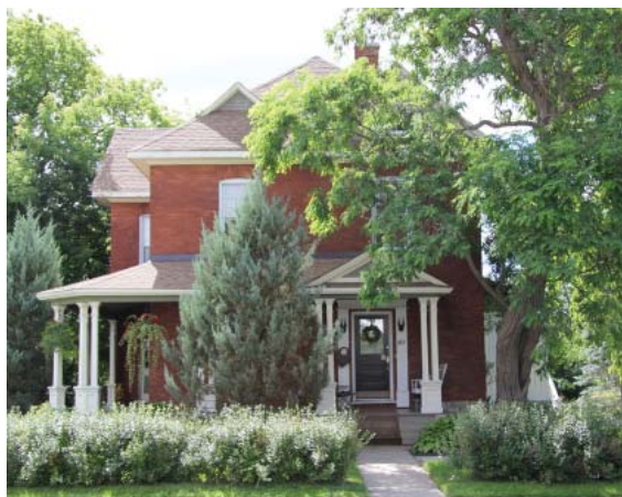
Example of a well-maintained wrap-around porch with paired wooden columns at 57 Main Street East. These decorative wood elements add character to the house and the District.
