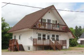
Example of post-modern style, on Queen Street.
