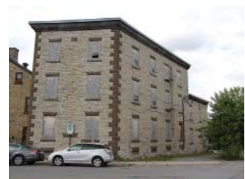
Former Almonte House Hotel in the Lanark Style.
