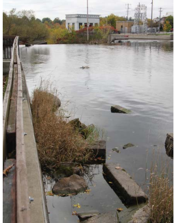
Relics and remnants of past industrial uses should not be removed without consideration and review.
